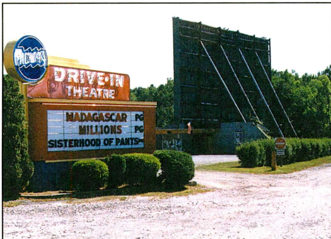
Midway Drive-In, State Route 48 in Minetto, New York. From the rear, timbers are used to support the giant screen. Some establishments place their FM transmit antenna atop the screen structure; others might affix an AM longwire to one of the logs. Like most of the very few remaining Mom & Pop local (often AM daytime-only) radio stations, most classic drive-ins are operated as a labor of love by true enthusiasts of the genre. Both are national treasures.
