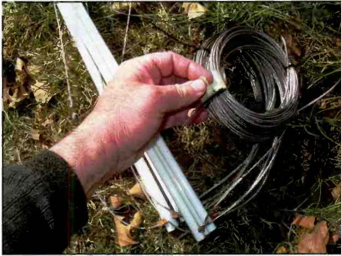
Carefully untape each roll of wire and extend the antenna. The entire process takes a few minutes, but it must be done with care and planning to ensure the wires uncoil easily.
