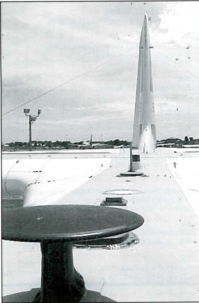
This photo shows the antennas on the top of the C130 when viewed from the escape hatch at the back of the cockpit. The big dish in front is the dual sitcom antenna with UHF and VHF. Behind it are the TACAN antenna, ADF No. 2 antenna and the UHF/VHF No. 2 communication antenna. And clearly seen is the high frequency Communication No. 1 antenna wires.
