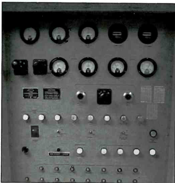
A close-up of a transmitter panel.
