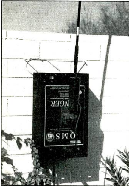
The "hidden wall" installation of the SGC coupler.
