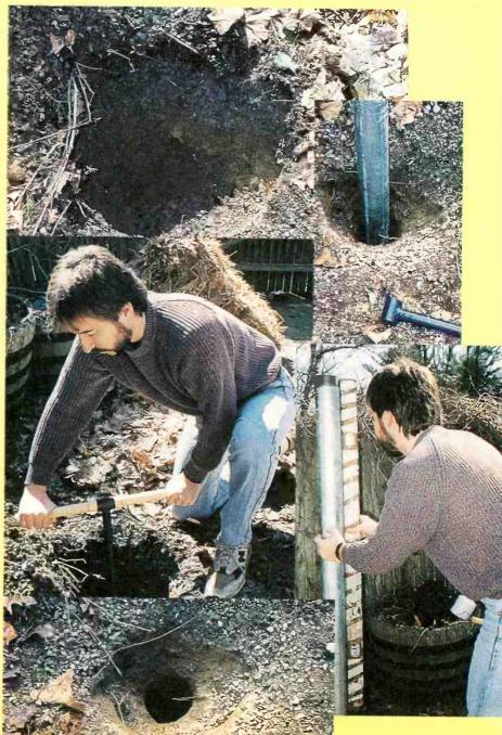
prevent the post from turning. Four additional metal pieces are attached to the clamps to act as guides for the Qik-Base's angle-iron "roots." Then the roots are pounded into the earth, the hole is filled, the sod is replaced, and you've got one sturdily mounted pole!
