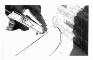
Fig. 2. Cement the wire into a groove in the sidewalk using some sort of construction adhesive.
