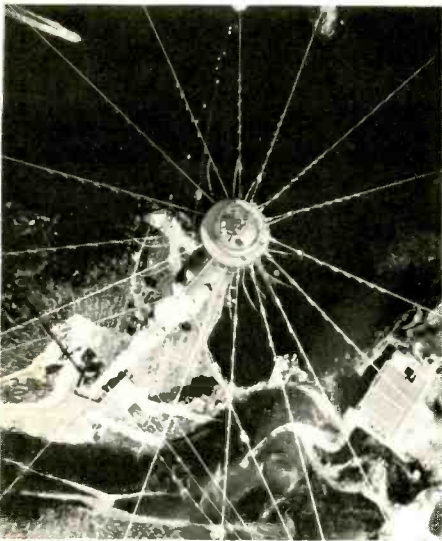
Two views of the 1500-foot antenna tower at OMEGA Station H in Tsu-Shima, Japan. Surrounding islands were used to anchor guy wires. Ten feet wide, the structure is tallest in Orient.
