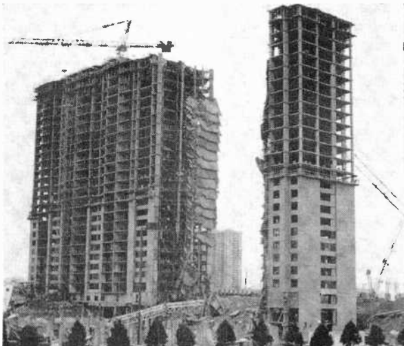
This is the site of the high-rise disaster, where a crane fell and brought down a whole section in the middle of the building under construction. Scene is Bailey's Crossroads in Virginia. Rescue operation was speeded by Fairco REACT.
