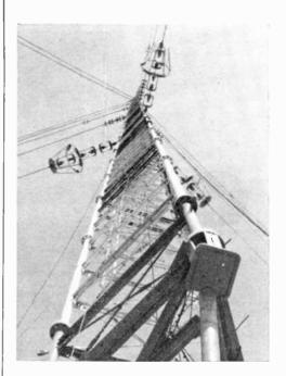
The towers are painted with alternate bands of orange and white to provide aircraft warning, though it is said that the steel's use would be enhanced if it were permitted to oxidize and form its own protective coating.
