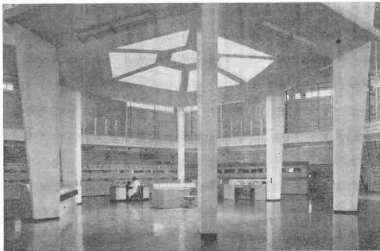
This is the impressive transmitter building of "Radio Vaticano," Vatican City.
