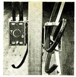
Front-to-back wiring technique is used by electricians to provide outlets to adjacent rooms. Conserve wire by running single downlead, and use a coupler.
