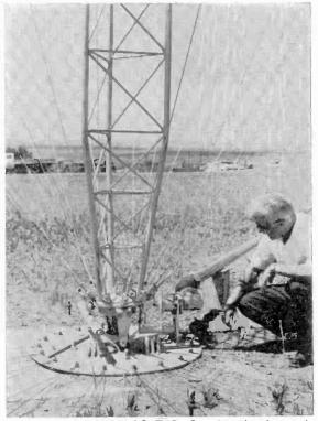
WWV RELOCATES—Construction is nearly completed on the new WWV transmitter building and control center at Fort Collins, Colo., from which the NBS standards broadcast station is scheduled to transmit beginning in December. Photo shows standby antenna fed by 31/8 " coax line.
