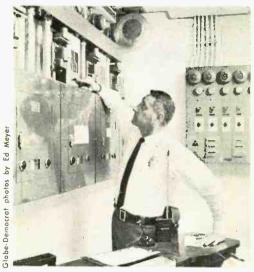
The office of Edward Thurman is headquarters for the Barnes security system. A transceiver on a desk is home base for the walkie-talkies, and a wall of alarms keeps watch for fires. Alarms also are linked to the "oxygen bank," set to go off if the oxygen supply dips low, and to the narcotics vault.
