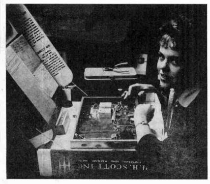
The contribution that kits have made to the hi-fi field can never be accurately estimated. Scott changed the kit building picture through use of color-coded wiring and pictorial diagrams.
