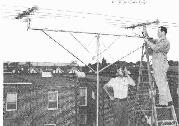
VERTICAL STACKING reduces fading
