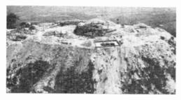
THE ENTIRE top of a mountain at Ajangote in Ghana, Africa, has been "decapitated" to make room for a high tower designed to support TV transmitting antennas, and buildings to house transmitting equipment. The elevation
