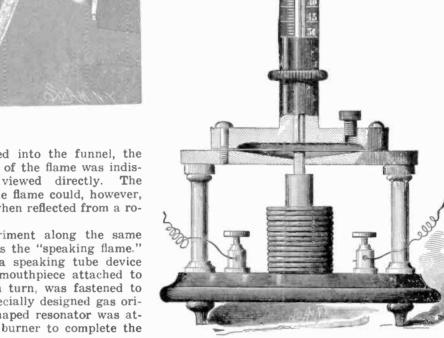
In crude ammeter above, current flowing through coil pulls a movable core down, activating a diaphragm and causing mercury in tube to fall. Device below is expansion voltmeter; it depends on linear expansion of a thin platinum wire when voltage is applied. Wire is coupled to pointer in front of scale.
