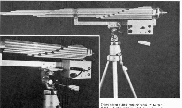
Thirty-seven tubes ranging from 1" to 36" make up the author's tubular mike; all construction details are given in text and in drawing at right. Completed unit is mounted on a camera tripod and panned like a machine gun to find sound source.
