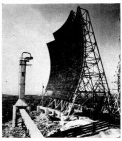
The \$5 million, 344-mile link provides 240 channels for voice communications and data transmissions. At Vancouver Island, a conventional 275-mile microwave radio system connects with the city of Vancouver and telephone circuits to the United States. The installation at tiny, storm-tossed Trutch Island, which is manned on a 24-hour basis, necessitated the formation of a community with all utilities for 27 people.
