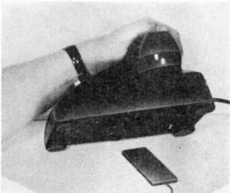
Flat type pickups can be placed under a telephone as above. By connecting the pickup to an amplifier, you can monitor family, business conference calls.
