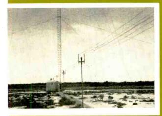
Three towers (one is shown above with its transmission line) are used in the highly directional Radlo Marathon antenna array. Signal in U.S. is weak.
