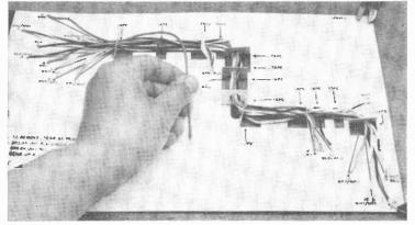
A jig or template is used to assemble the A50K's chassis wiring harness. Tie wires hold harness in shape as it is dropped into chassis. Leads are colorcoded and offer a neat and orderly way of getting connections from front to rear of chassis without creating a "rat's nest."
