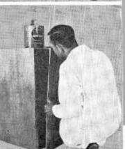
Plywood sides are glued but not nailed in place. Depending on the type of cement you use, it may be necessary to apply some pressure while the cement is setting.
