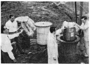
Generator for power station is lowered into half-buried cylinder during tests at Baltimore, Md., plant of the Martin Company. Unmanned station will operate without maintenance or refueling for two years once it is completely assembled and fully sealed.
