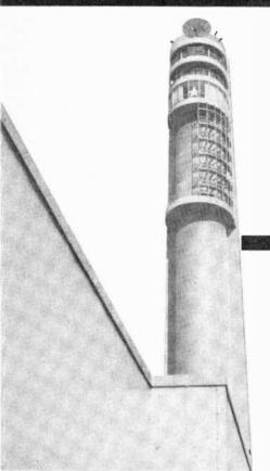
This ITT tower in Nutley, N. J., is used for microwave experiments. To prevent the possibility of dangerous radiation, a trapdoor interlock shuts down the transmitters whenever a technician goes on the roof to service the antennas.
