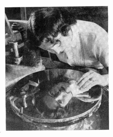
Infrared "picture window" produced by scientists at Hughes Aircraft is solid germanium casting 15" in diameter and ½" thick.
