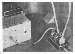
screws; connect one end of a length of lamp cord to the receptacle, and attach a male plug to the other end. Be sure not to overload the wall socket or receptacle with appliances draining more than either one can handle.—Art Trauffer, Council Bluffs, Iowa.
