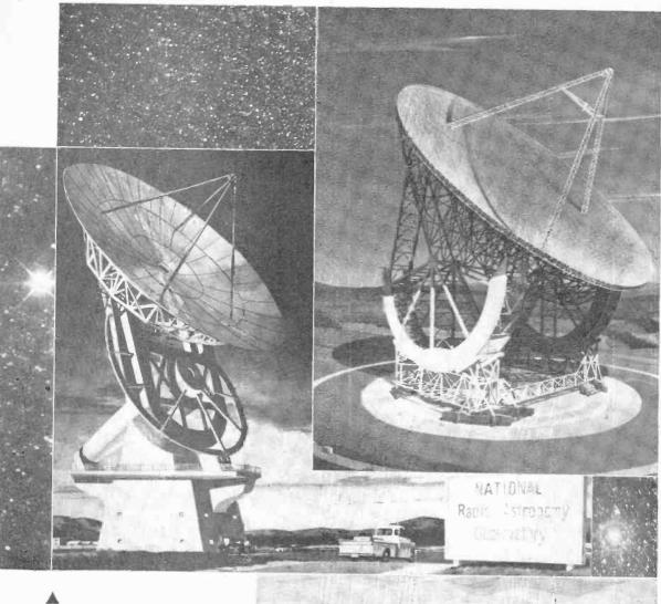
Under construction at the National Radio Astronomy Observatory in Green Bank, W. Va., is this 140' precision telescope. The surface of the reflector will be more than one-third of an acre in area and is designed to be accurate within a quarter of an inch. When completed, the 210'-high instrument should be the most highly accurate radio telescope in the world.
