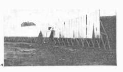
Primary reflector of radio telescope at the Pulkovo Observatory in Russia looks more like a board fence than a scientific instrument. Each panel is about 4' by 10' and can be adjusted individually. The 425' multi-paneled reflector directs all energy it receives into a much smaller secondary reflector located 200' away at the focus of the primary reflector.
