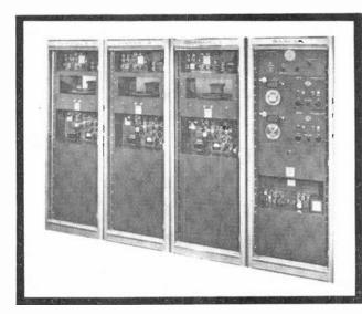
Transmitter racks for the wired pay-TV system. Each of three channels (A, B, and C) carries not only a program, but also the price information and code numbers to identify the program. The fourth ("Barker") transmitter carries a recorded message which announces up-coming programs.
