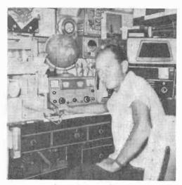
Anson Boice. WPEIBD, works with a Hammarlund HQ-100 and a Grundig receiver. His current equipment also includes a Webcor tape recorder and a POP'tronics antenna tuner.
