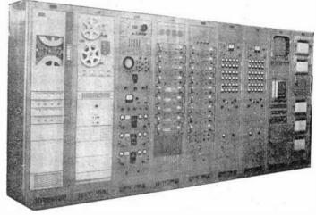
nals which are demodulated, sorted out, and turned into understandable form. In some cases, the signals are decoded as fast as they are received; this is called "real-time" telemetering. Most of the information is recorded by tape recorders for later study. Some advanced telemetering systems feed selected information directly into computers for immediate processing, as mentioned above, making it possible to notify a pilot of danger developing before he is aware of its presence.
