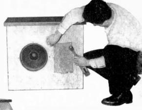
8 Plastic hi-fi grille cloth made by Mellotone is wrapped around cabinet and stapled into place. This material is recommended for speaker enclosures because it is strong, goodlooking, and acoustically transparent. After the grille cloth is stapled, legs or a base can also be installed.
