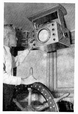
**Ceiling radar installation** saves space and allows shorter lead-in cables to antenna atop wheelhouse. (RCA photo)
