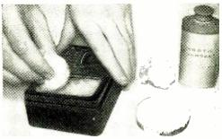
cular motion. After the scratches disappear, apply a daub of toothpaste to some cotton or felt, dip it in water, and use it to finish buffing.—Charles A. Lang, San Francisco, Calif.
