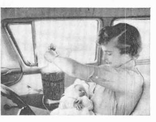
Electronic bottle cooler-warmer, with no moving parts, plugs into car's cigarette lighter. Fifty thermoelectric junctions cool or heat the bottle instantaneously. The current that produces cold can be reversed to produce heat for cooking. This experimental Westinghouse device has vertical aluminum fins for air cooling or dissipation of removed heat.
