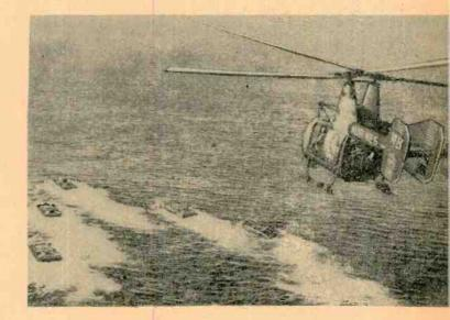
A wave of Marine Corps amphibious assault vehicles churns toward the California coastline under the electronic control of the operator in the helicopter. The radio control system was developed to put the vehicles through rugged surf tests without endangering human lives.
