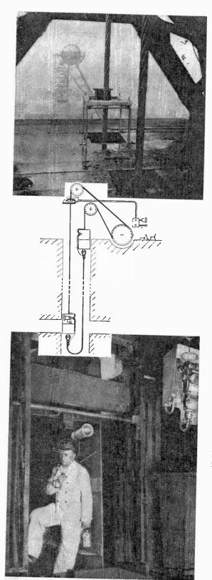
possible failure of an ordinary telephone communications system between a mine head and shaft, a German engineering firm, Standard Elektrik of Stuttgart, has switched to a new method using the elevator hoisting cable as the secondary "winding" of a transformer.
