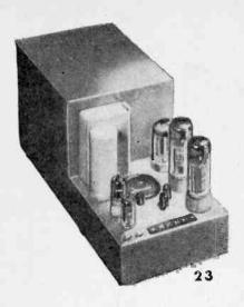
Using same basic design as larger model, this 30-watt power amplifier employs an "Ultra-Linear" circuit, terminal board construction, a meter indicator for tests and adjustments of bias setting. Marantz Model 5.
