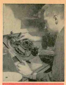
Start of test procedure consists of a visual check and final settings of parts fits and clearances. Changer is mounted on special "flip-over" fest stand. The tester sets height of tone arm, checks smooth operation of pivots, and adjusts velocity trip friction so that change cycla actuates only after the last groove of the record. Also, stylus pressure is set for all changers.
