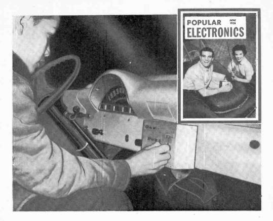
MANY PEOPLE want to know if it is possible to purchase a portable radio and operate it in an automobile as well as take it on a picnic. It is possible. But the portable would have to be built in a metal case to shield it from the ignition system. And inasmuch as the metal car top and body would prevent the radio waves from reaching the built-in antenna of the set, an outside antenna must be installed.
