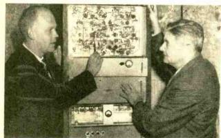
A TOMIC MOVEMENT is used as the world's most accurate time standard in the new "Atomichron" clock, shown at left with its creators, Dr. Daly of the National Co., Malden, Mass., and Dr. Zacharias of M.I.T. Far more accurate than the pendulum of crystal-controlled timing devices, the "Atomichron" varies by no more than one second in 3000 years. Here, atoms control the frequency of an oscillator circuit.
