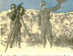
Sparing themselves uncertain journeys to nowhere, weathermen later developed ways of charting balloon flights from the ground. Above, an optical instrument—called a theodolite—tracks the balloon after it is released by the soldier holding it, thus recording speed and direction of upper winds.
