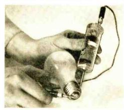
with a nut. Push the dry cell down in the bottle until it makes firm contact with the head of the brass screw. The screw's pointed end serves as one of the test points.
