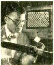
square inch of glass contains 250,000 holes, or cells. Information is "written" into the cells by an electron beam scanning the screen. Another beam "reads" it.
