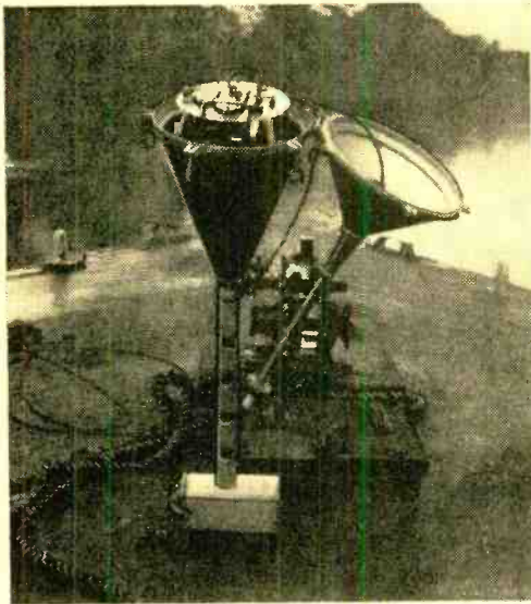
Floating transmitters are read out for whaling fleet (above) to signal location of floating whales killed by catcher boats to the factory ship which gathers them in. Transmitter is shown on buoy at left.
