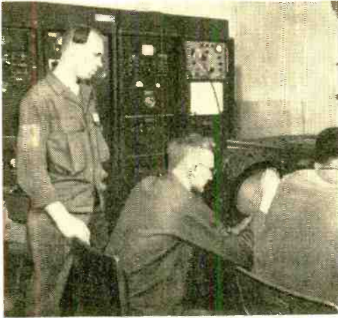
Electronic equipment shown above is installed in one of the gap-filler radar stations which are located between more powerful long-range search transmitters.
