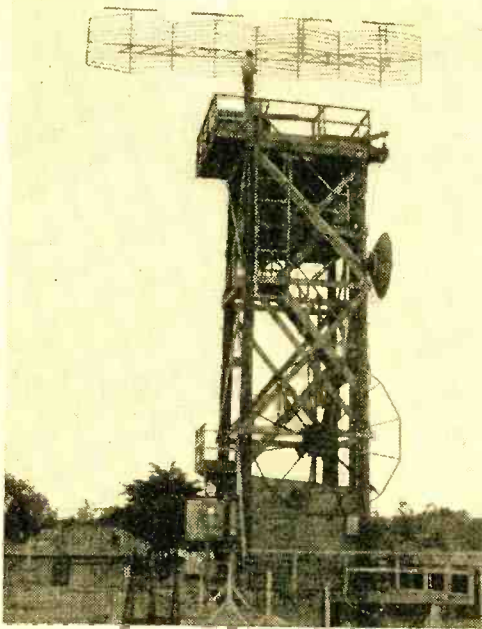
Meteoric effects on long-range TV reception are being studied at Stanford University with the assistance of this huge TV-type antenna.
