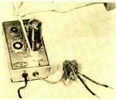
a suspected tube placed in the proper socket. A good heater will cause the neon lamp to glow. Another pair of wires lets the neon lamp test tubes or special equipment independently of the sockets.
