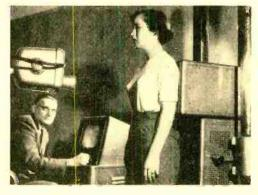
Amplified light provides clearer, brighter x-ray images, and makes possible fluoroscopic examination in a lighted room (above). At right, Ralph E. Sturm, co-inventor of the Lumicon demonstrates how the device might be used to inspect luggage. April, 1956
