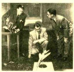
Using electronic records salvaged from jet plane, NAA engineers recreate its position and probable movements just before crack-up.
