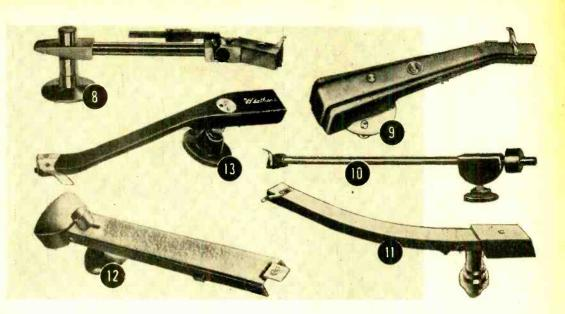
rest. Resonance is said to be beyond audible limits. Device was designed by D.T.N. Williamson of amplifier fame. Entire suspension is located beneath the mounting platform. Safety device prevents damage to record or stylus if arm is dropped accidentally. Complete system net, \$75.00 (approximately). Ferranti Electric, Inc., 30 Rockefeller Plaza, New York, N.Y.
