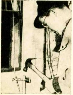
In this case, make a "ground" by driving a pipe or ground rod four or five feet into the earth. Connect the ground wire to the pipe with a clamp.
