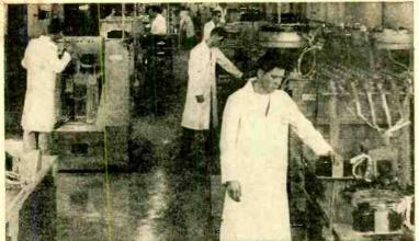
Machines make ceramics, process and apply parts to wafers, assemble modules, and perform complete inspection.
