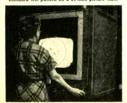
In place in a home receiver chassis, the picture tube is checked before the completed unit is installed in a cabinet. Unit around neck of tube deflects electron beam to sweep the screen.
