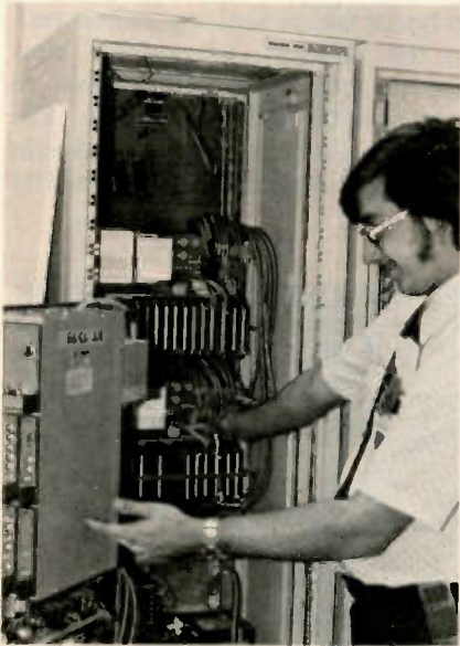
Figure 7 A technician opens an X-ray generator in preparation of inspection and callbration.
