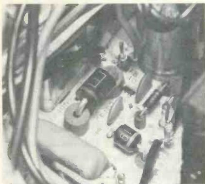
Figure 2 Three diodes of different sizes are almost hidden in the wires between the pincushion-transistor heat sink and the flyback (at right). The smallest diode is CR403 which rectifies the +210V supply. Below it is the medium-sized CR401, and the large CR402 is shown at the left.
