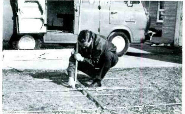
3:04 pm The antenna is pulled from its box, the elements are unfolded, and the antenna is layed out on the ground (or driveway if the lawn is wet or muddy). Next, the 4' rotator mast is attached to the antenna.
