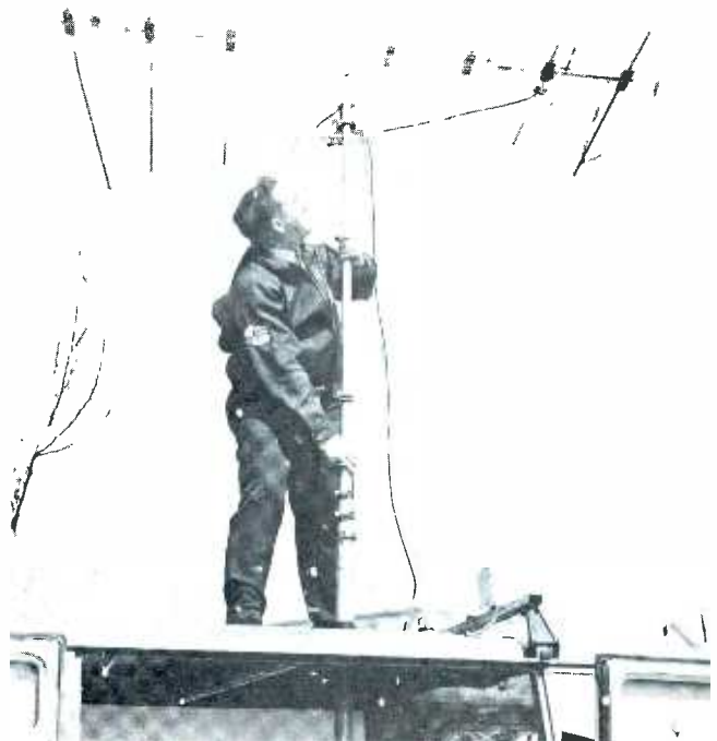
Fig. 9. Elevating the antenna, one section at a time.
