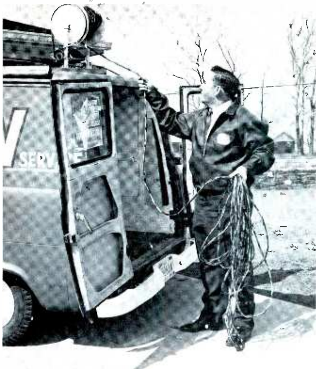
Fig. 8. Pulling the cable from the storage reel.
