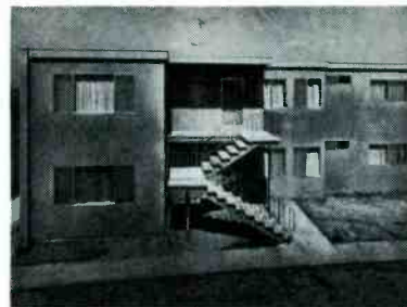
Another Wizard 300 Master Antenna System — one antenna — 12 outlets — no amplification—done entirely in twinlead. The Towne Apartments, Downey, California.
