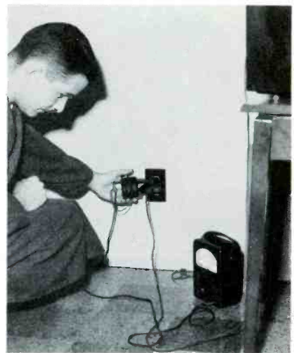
Fig. 7. Checking line current with line separator and clamp-on adapter.
