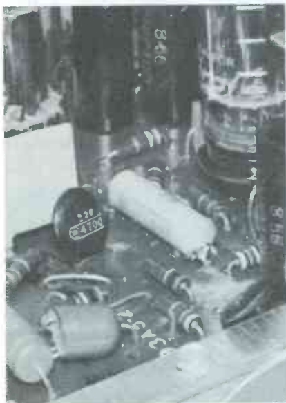
(B) New capacitor in circuit.
