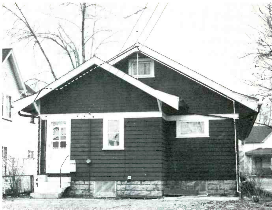
Fig. 4. This end view of a house shows the system of wires and ground rods necessary for secure grounding of an antenna system.
