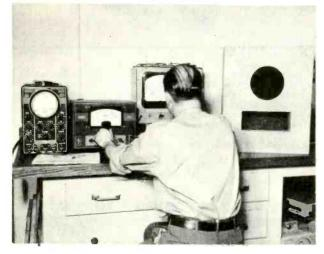
Figure 1. Equipment Used in Determining Resonant Frequency of Speaker and Data for Impedance Curves.
