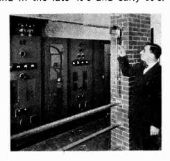
A large pre-war FM station, W43B, Paxton, Mass. This station transmitted on 44.3 MHz with an effective radiated power of approximately 300,000 watts. It covered most of southern New England.
