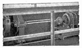
FIG. 6.880.—Euclid crane construction 7. Bridge drive mechanism. The illustration also shows the motor mounting between the bridge motor and the gear housing.
