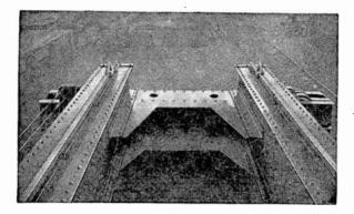
FIG. 6.875.—Euclid crane construction 2. Gusset plates. These are used to the the girders to the end trucks, making it impossible for the crane to weave and get out of square on the runway.
