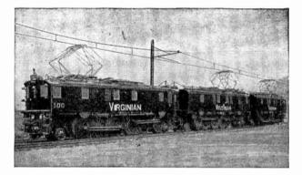
FIG. 6,117.—Westinghouse equipped, single phase, 215 ton motive power units as used on Virginian Railway.
