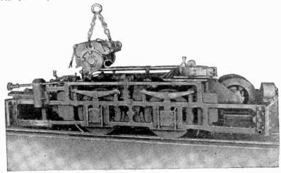
FIG. 6,177 .- Method of removing top haif of split frame motor and armature.
