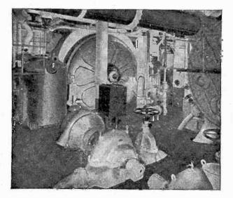
FIG. 7,171—Propelling motor and condenser pumps of S.S. California quadruple screw turbine electric drive; General Electric equipment,
