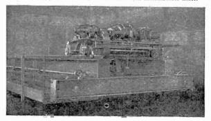
FIG. 6,879.—Euclid crane construction 6. End truck construction and driving side of the crane trolle. In design the line shaft, bearings are closely spaced.
