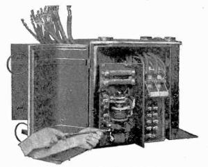
FIG. 6,297 .- Westinghouse control operation 9. Adjusting type 371 overload relay.
