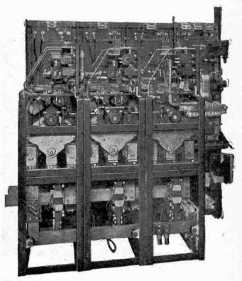
FIG. 7,178-Rear view of General Electric control panels for Ward-Leonard or variable voltage control.
