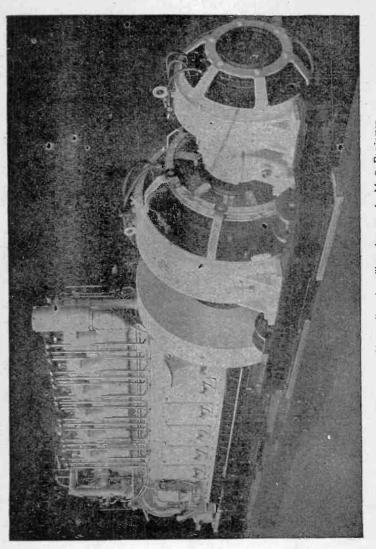
FIG. 7,179,--General Electric Diesel engine with main and auxiliary dynamos for M. S. Farrington.
