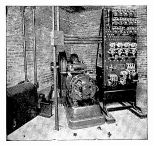
FIG. 6,820.—Cutler Hammer full magnetic, single speed push button d.c. controller panel installation showing clevator machine. When push button control is used the car is sometimes "stolen" before the person in it has had a chance to open the car gate or door after arriving at its destination. To overcome this objection a non-interference relay may be used to provide ample time for opening the gate or door.
