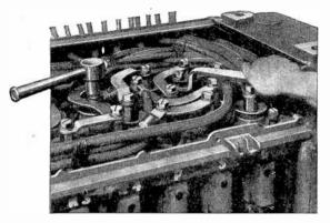
FIG. 6,274.-Westinghouse control operation 3. Tightening terminal bolts.
