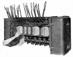
FIG. 6,277.-Westinghouse control operation 4. Removing arc boxes.
