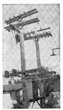
Fig. 8,435.—Westinghouse resonant control installation as applied to series lighting circuits.
