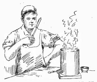
Fig. 8,628.—Method of judging the heat of a soldering bit or so-called "iron," illustrating sensible heat.
