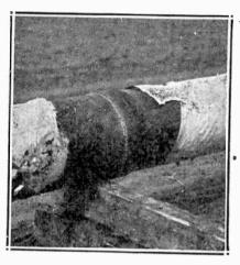
Fig. 8,171.—Typical burning-in weld in a plain and spigot joint.
