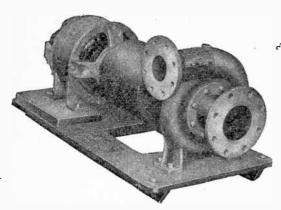
rig. 8,795. — Fitz Rualite turbo-generator set comprising a completely self-contained hydro-electric power unit, including Fitz high speed water turbine direct connected to electric generator and provided with built in automatic governor. Scandard units available in capacities ranging from 32 kw., capacity to 100 kw. capacity.
