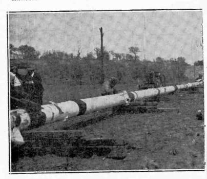
Fig. 8,169.—Section of pipe line being welded. Note the use of wood skids for blocking up section so that it is level. Photographed on Texas Pipe Line Company's Monahans-Port Arthur, Texas, line.
