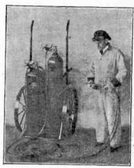
Fig. 8,146.—Lighting the acetylene. Open the acetylene needle valve on torch and light torch with a spark lighter.
