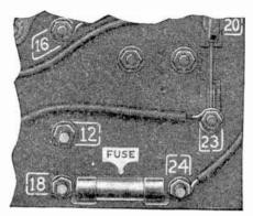
Fig. 8,788.—Delco automatic direct lighting plant control. 7. Fuse. If at any time the plant fail to start, examine the fuse which is mounted on the back of the switchboard. Do not use a larger ampere fuse than the one that comes with the plant or is recommended by the factory.
