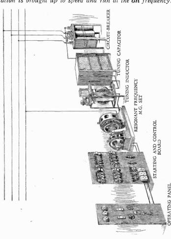
Fig. 8,434.—Westinghouse resonant control station equipment, three phases energized consecutively.
