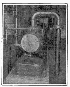
$F_{1G}$ . 8,188.—Gas compressor installation showing welded joint tube turn fittings in suction and discharge connections.
