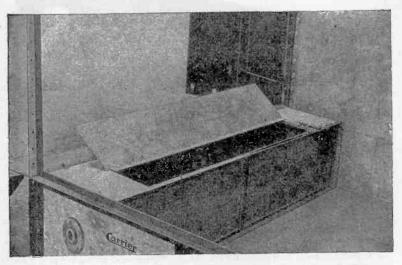
Fig. 8,759.—Carrier fixed suction strainer, the cover open. The pump connection shows in the lower left corner.
