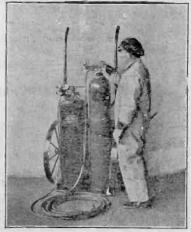
Fig. 8,140.—Connecting the hose to the regulators. (Airco-Davis-Bournonville.) Connect Fig. 8,141.—Opening the cylinder valve. (Airco-Davis-Bournonville.) Release regulator
