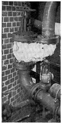
Fig. 8,193.—Pennforge butt welding flanges. View showing installation of these flanges in the Harvard University power house.
