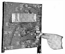
Fig. 8,789.—Delco automatic direct lighting plant control. 8. Service switch. The small knife switch that is located on the back of the switchboard should be opened only when cranking the plant by hand. When the plant is running, the switch must be closed. The plant will not start automatically while the switch is open.
