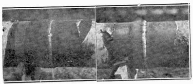
Fig. 8,172.—Pipe line joint showing portions of burning in weld and finish weld in a plain bell and spigot joint. Photographed on Texas Empire 600 mile line.
