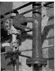
pressure, 150 lbs. have plain or raised faces, as ordered. Flanges for higher pressures have raised faces. Fig. 8,191 shows the general appearance of a butt weld pipe flange.
